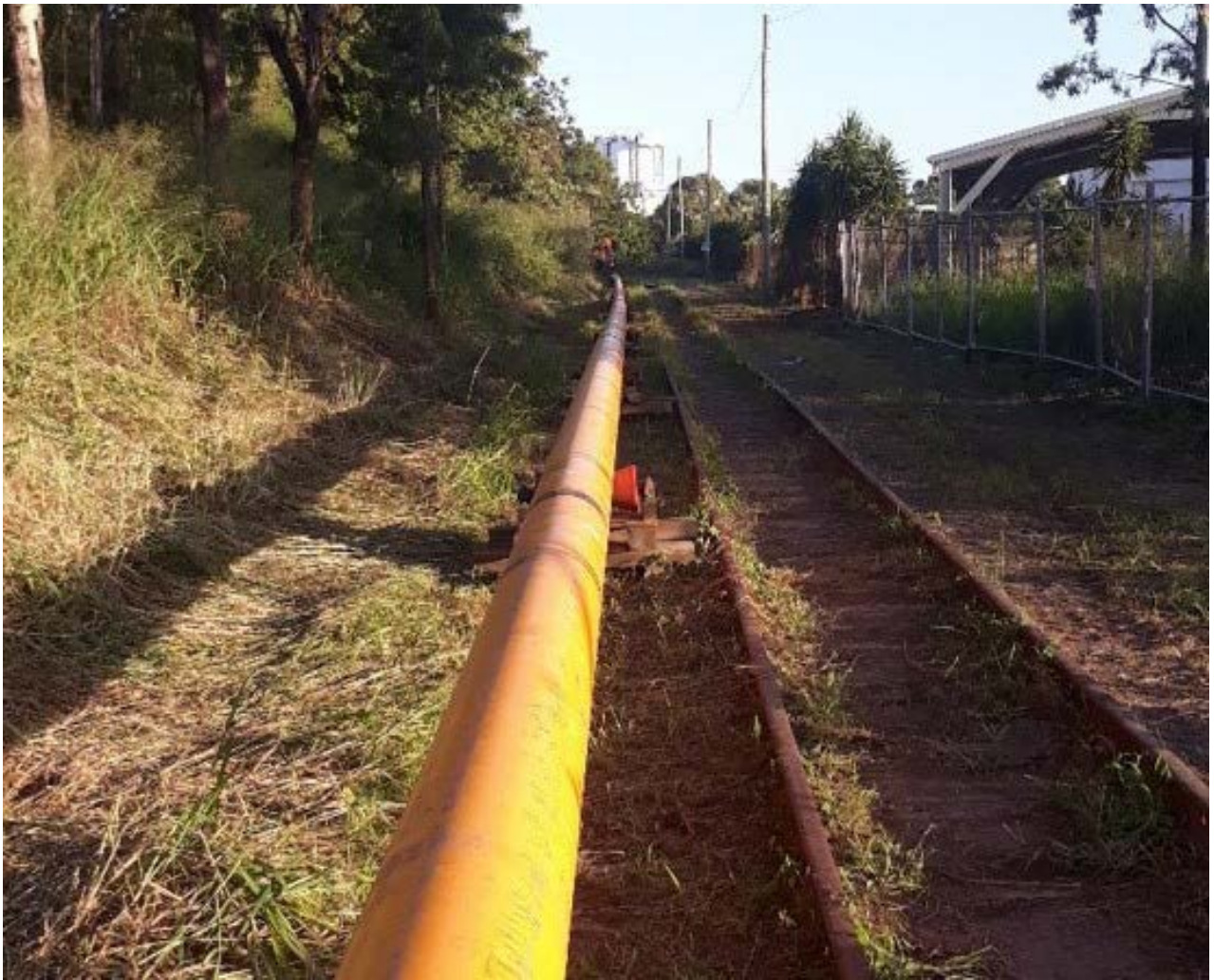
Figure 4.1 The right of way used for the HDD sting construction
