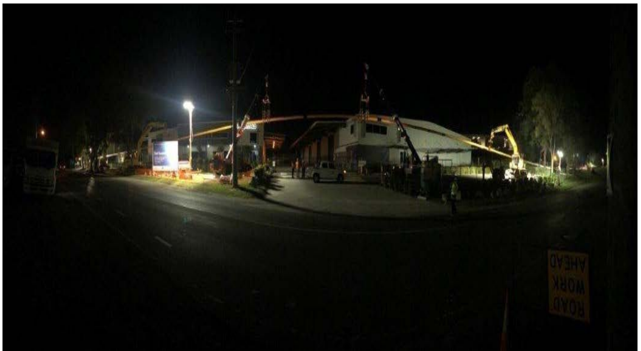
Figure 4.2 Sting elevation over commercial drive during pull back activities
